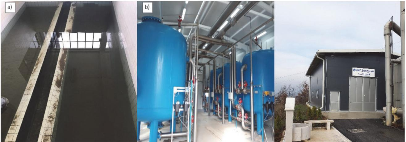
Figure 3. Filters situated in Karašnica plant: a) gravity filter b) filters under pressure and facility accommodating these filters
