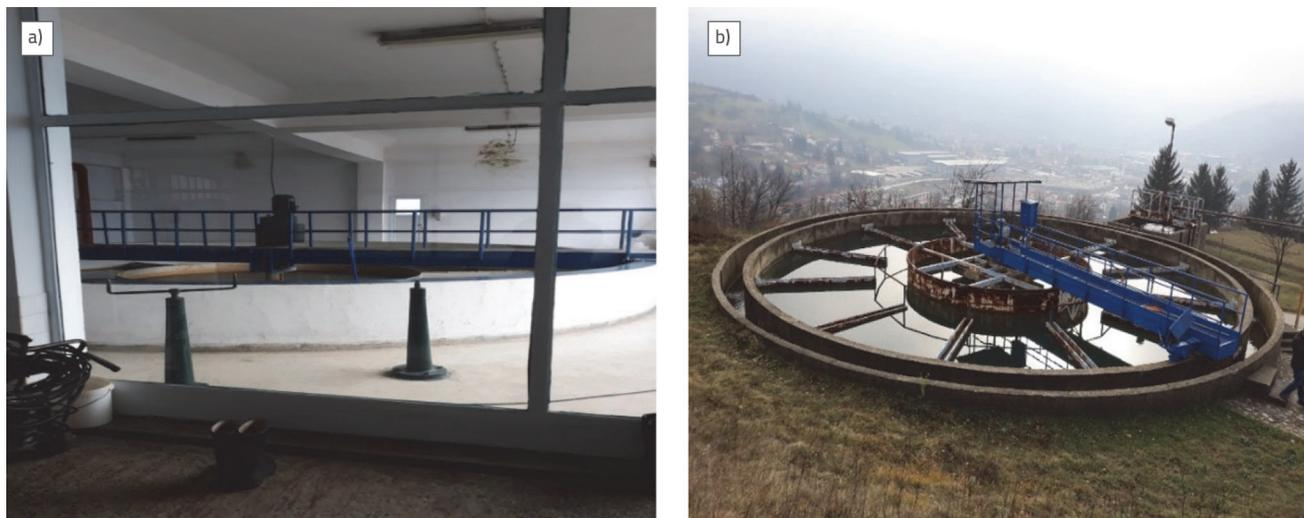
Figure 2. Circular settling tanks at Karašnica plant: (I) internal settling tank (T1) with a capacity of 50 l/s (II) external settling tank (T2) with a capacity of 100 l/s
